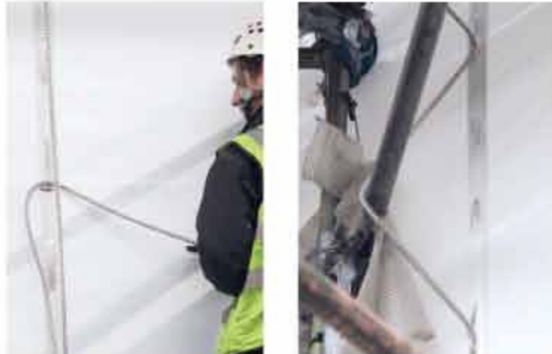
Single sided PVC Coated Weldable Webbing with built in attachment loops. Huge time savings in construction and material. No dragon tails required.
